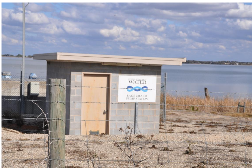
Figure 5.9 Lake Charm Pump Station
