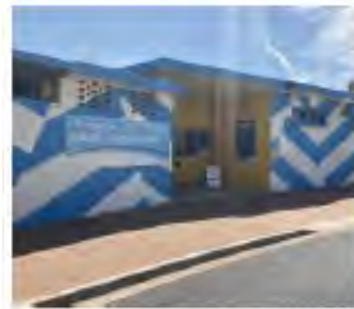
Outdoor pool entrance
