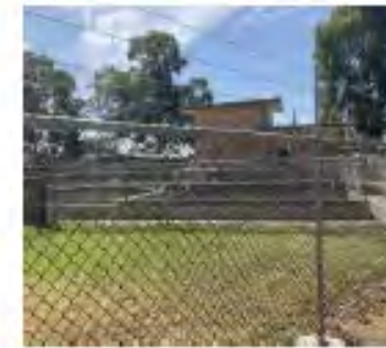
Ageing plant room
