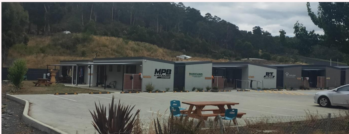
Image: Example of backpacker and seasonal worker accommodation in Huonville, Tasmania
