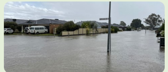
Photos: Flooding outside the Murrabit Hall (top), Kerang Swimming Pool (middle) and the intersection of Brolga and Marne streets, Kerang (bottom) following rain on Christmas Day 2023.
