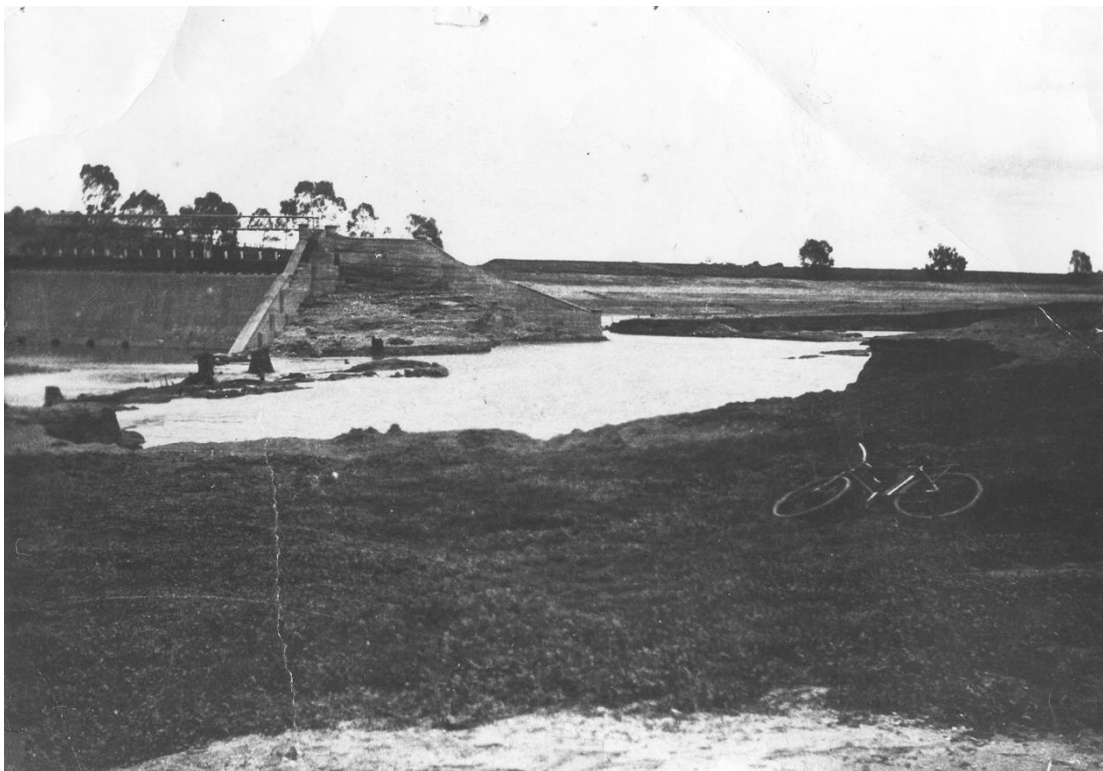
Picture above: Laanecoorie Reservoir Dam Wall Failure, 1909
