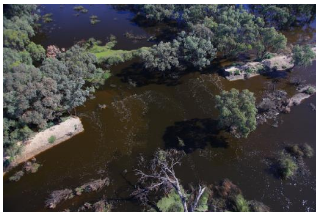
Photo above: breach in the Lower Loddon Levee, Jan 2011 Flood (photo courtesy North Central CMA)
