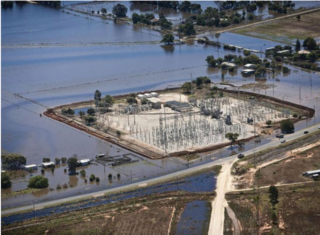
Left: Aerial view of Kerang Power Sub-Station in 2011. A permanent levee constructed around the Kerang Power Sub-Station successfully protected this critical infrastructure in 2022.
