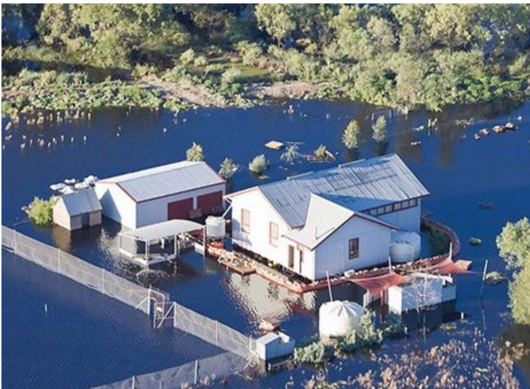
Left: Aerial view of Benjeroop Public Hall in 2011. A permanent levee constructed around the hall successfully protected the hall in 2022 and provided a safe location for the community.
