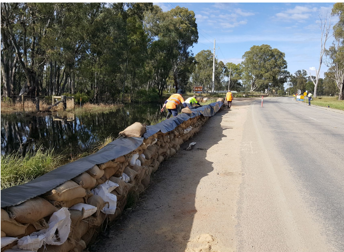
Left: Constructed temporary levee Koondrook October 2022
