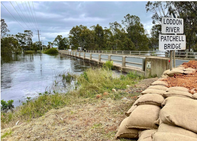
Above: Patchell Bridge over Loddon River Kerang, Oct 22
