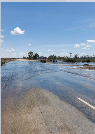
BELOW: Wandella Creek inundated the Murray Valley Highway at Reedy Lake, north of Kerang.
