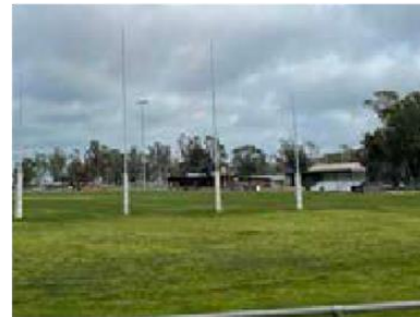
View across the main oval to pavilion and grandstand
