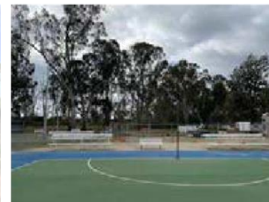
Recently resurfaced netball court and new agricultural society building under construction
