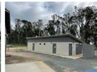
Recently constructed netball change and toilet facilities
