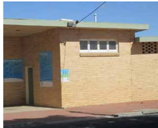
Replacement of barge and fascia timber
