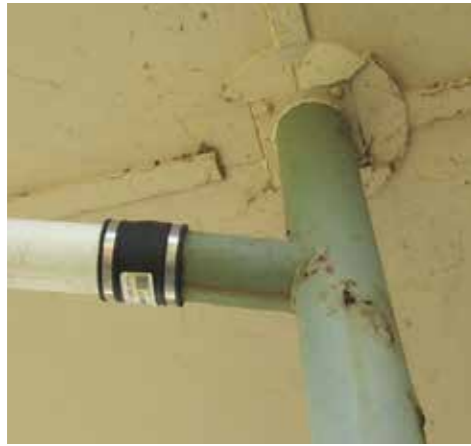
Replacement of Structural members where required.
