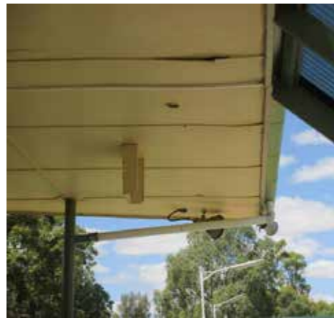
Removal of fibre-cement ceiling lining, very likely containing asbestos
