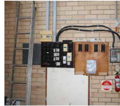
Replacement of existing switchboard located in office & first aid
