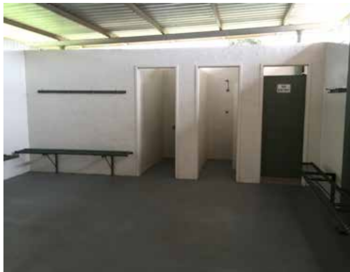
Upgrading of existing change area Including; New Floor and wall surfaces New seating, hanging rail, and Lockers New Lighting
