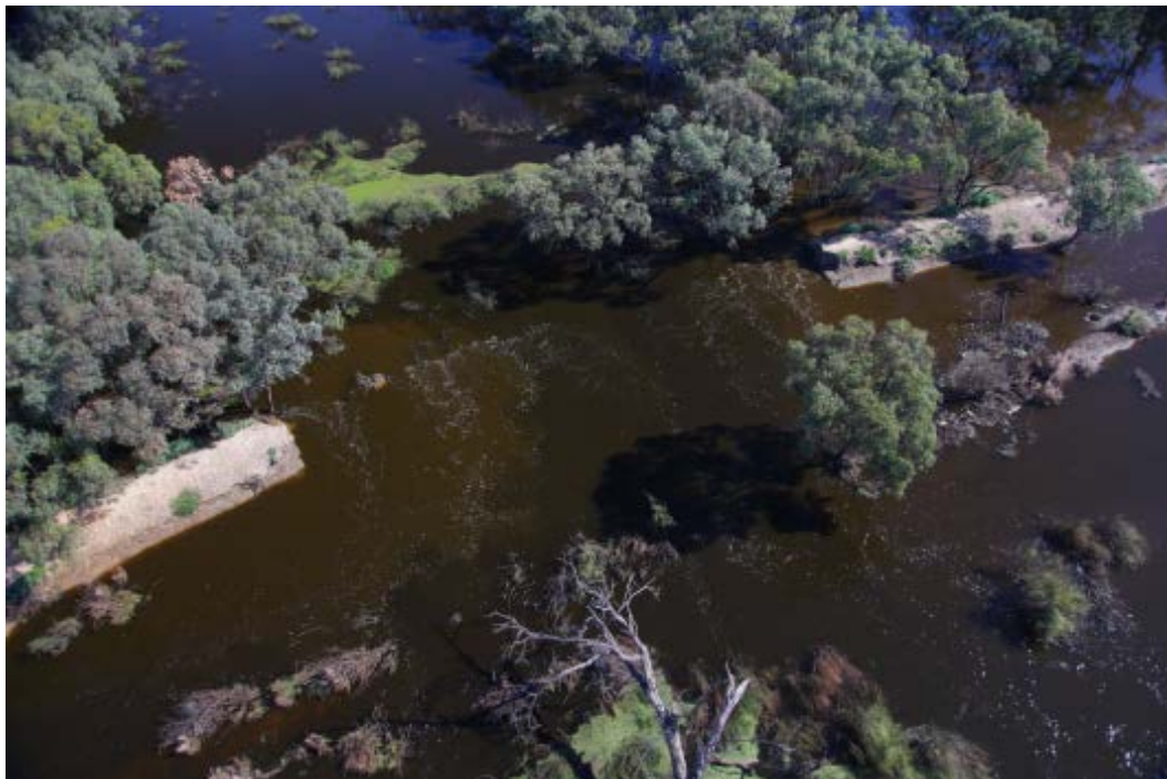
Photo above: breach in the Lower Loddon Levee, Jan 2011 Flood (photo courtesy North Central CMA)
