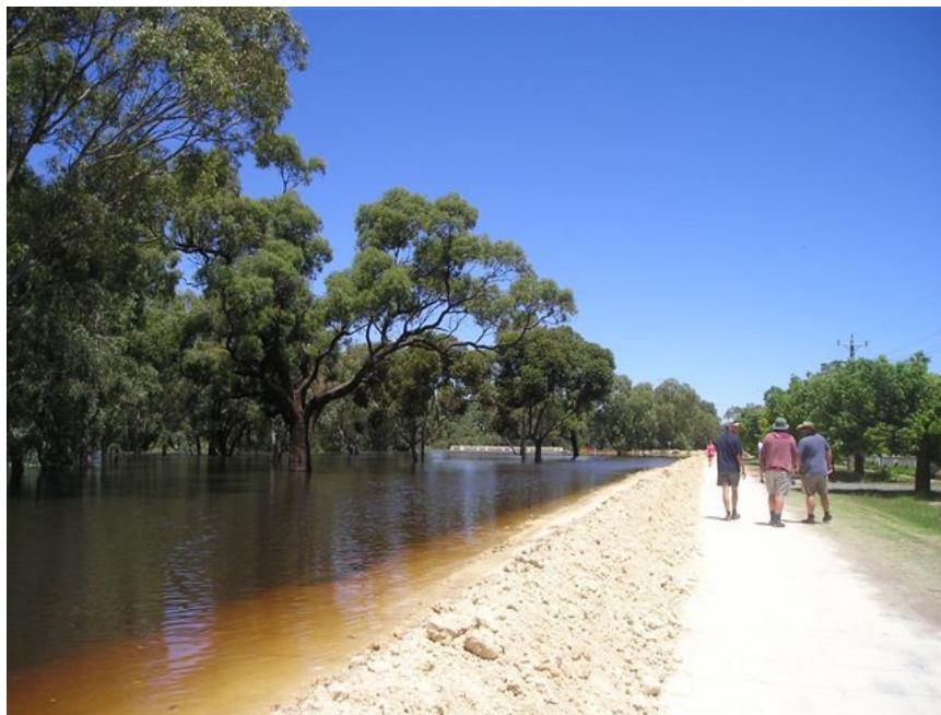
Picture above: temporary Works at River Street, Quambatook in January 2011 (photo courtesy Gannawarra Shire)
