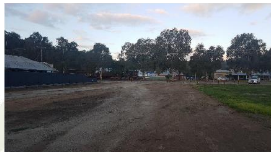
Figure 8 Site towards Main Street
