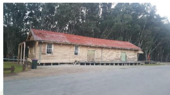
Figure 12 Former railway building/proposed restaurant
