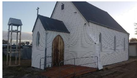
Figure 7 Existing church on site
