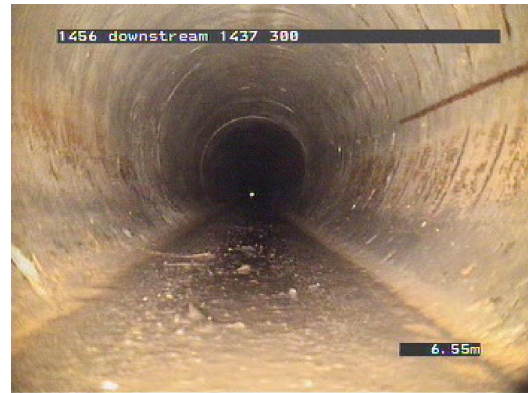
Figure 2-13 - Exposed circumferential and longitudinal reinforcement. Also note sediment build-up. Conditions rating 7 to 8 (Pipe 1456-1437).
