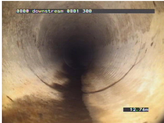
Figure 2-11 - Circumferential crack from 3 to 9 o'clock Condition rating 5-6 (Pipe 0800-0801).
