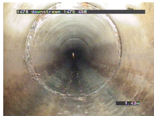
Figure 2-9 - Minor spalling concrete at joint. Condition rating 3 to 4 (Pipe 1478-1475).
