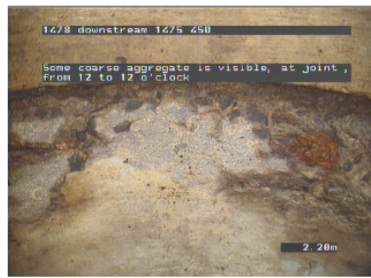
Figure 2-10 - Close view of spalling defect in Figure 2-9.
