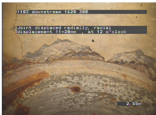
Figure 2-12 - Greater joint displacement, spalling concrete and cracking. Condition rating 7-8 (Pipe 1183-1620).
