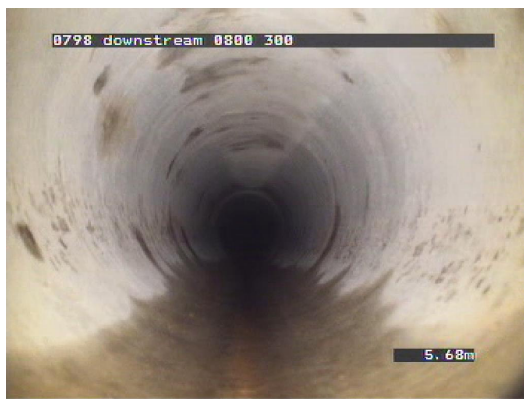
Figure 2-7 - Good pipe condition. Condition rating 1 to 2 (Pipe 0798-0800).
