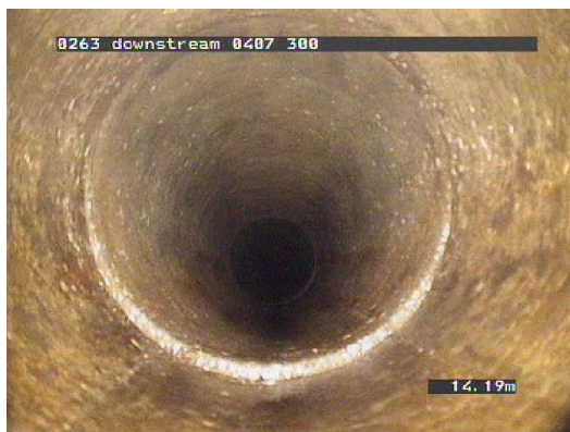
Figure 2-8 - Minor joint displacement. Condition rating 3 to 4 (Pipe 0263-0407).
