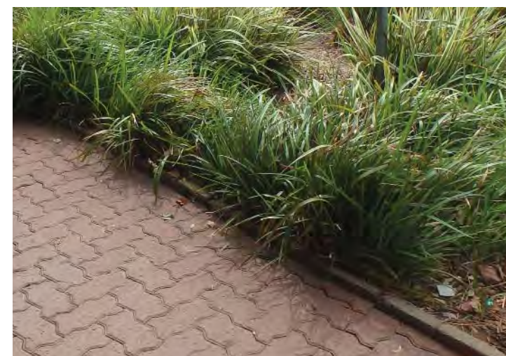
Example of paver edging to garden beds to the north of Victoria Street.
