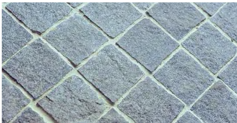
Traffic calming bluestone cobbles (approx 100mm x 100mm x 40mm)
