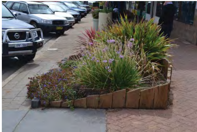
Wooden Garden bed cut into sloped footpath surface, with degrading timber edge.
