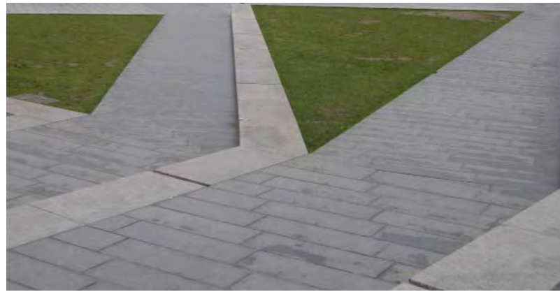
Concrete pod edging
