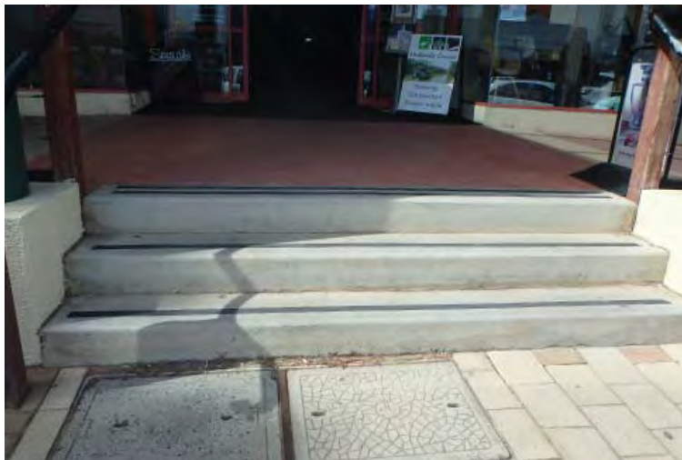
Steps to Patchell Plaza entrance.
