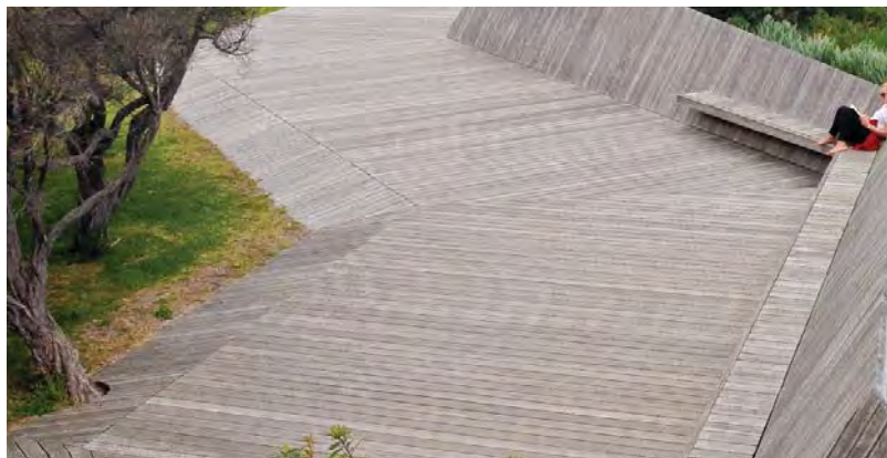
Timber deck with incorporated ramp.
