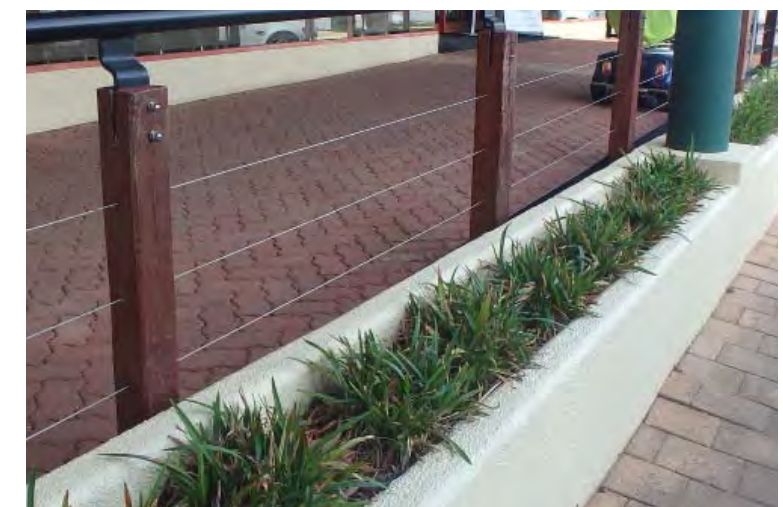
Good condition of interlocking paver adjacent to Patchell Plaza.
