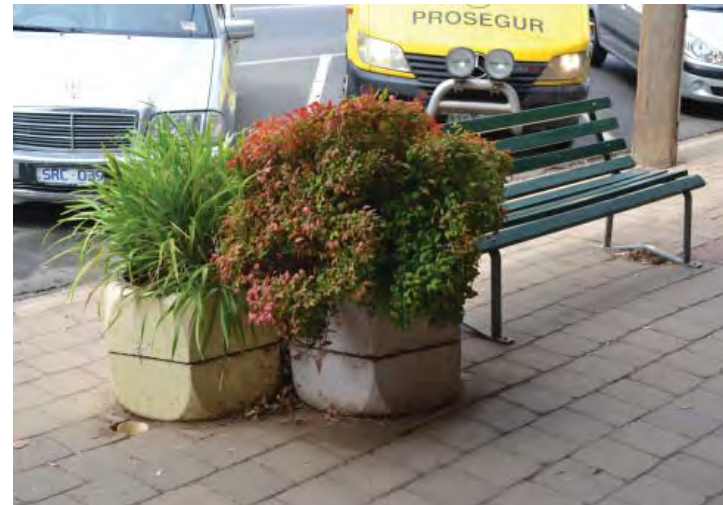
Irrigated concrete squared pot planters, with flaking coloured paint.
