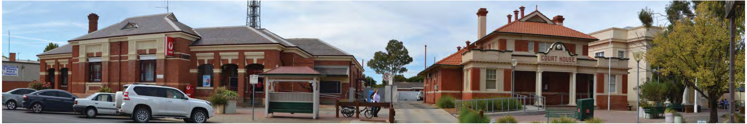
View of historically significant buildings within background of Victoria Square including the Courthouse, Municipal Building and Post Office.
