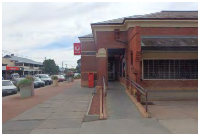
Ramp entry to Post Office from Victoria Square.
