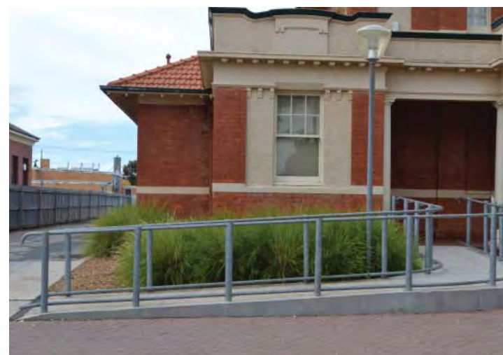
Ramp structure to Courthouse frontage.
