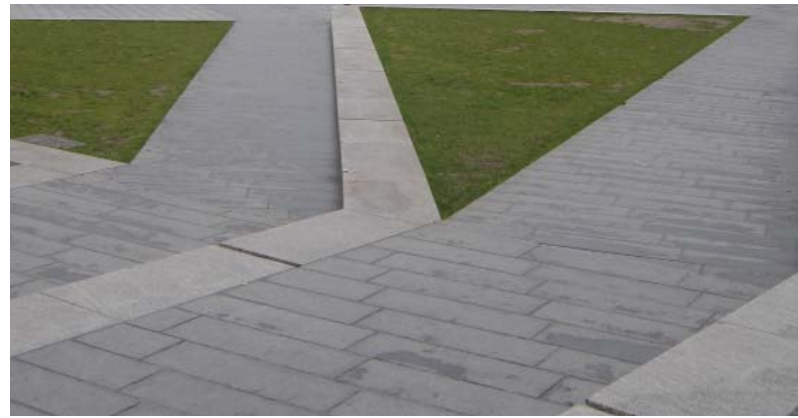
Concrete pod edging
