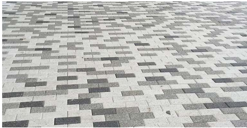
Coloured Concrete pavers - grey tones (approx. 600mm x 300mm x 40mm)
