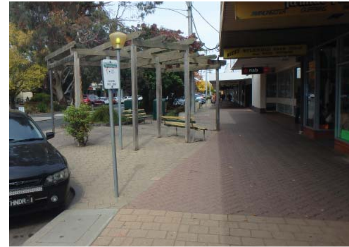
Mixture of pavement types within centre of Victoria Street.
