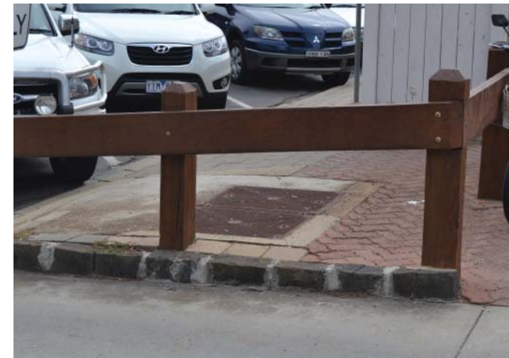
Bluestone edging to Victoria Police crossover adjacent to Victoria Square.
