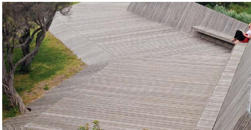
Timber deck with incorporated ramp.
