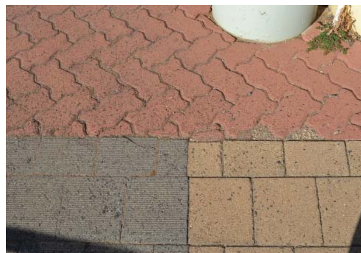
The three most common paver types along Victoria Street: yellow and grey concrete unit pavers and red interlocking pavers.
