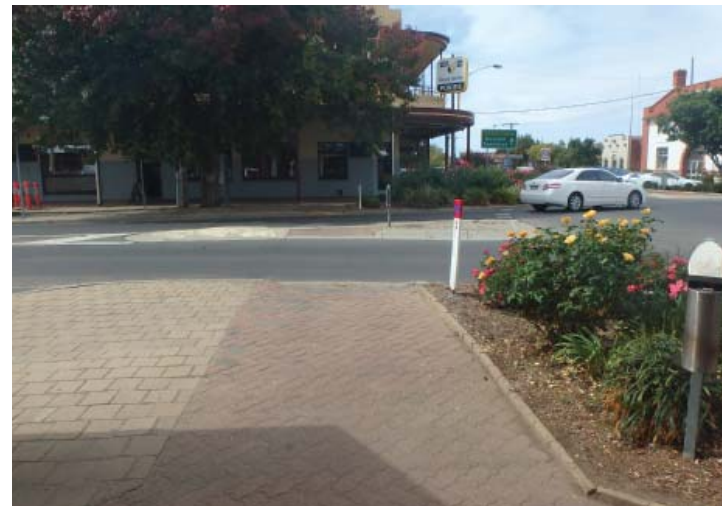
Interlocking paver extending to pedestrian refuge within road reserve.
