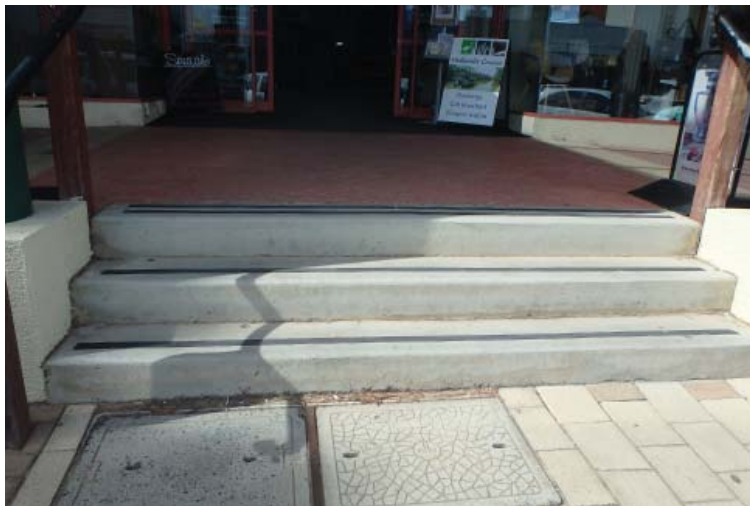
Steps to Patchell Plaza entrance.
