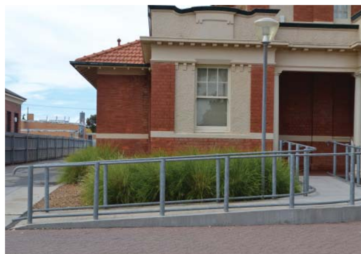
Ramp structure to Courthouse frontage.
