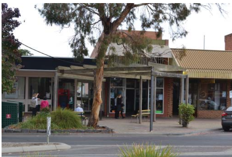
Arbor structure opposite Victoria Square, with damaged upright supports.
