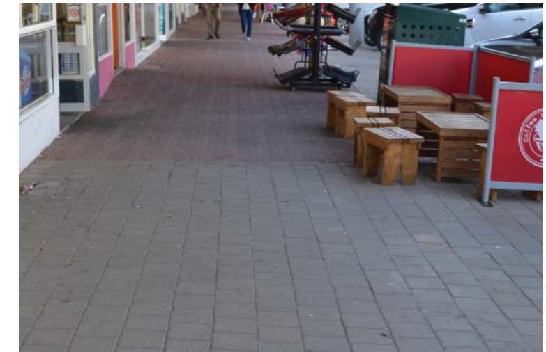
Uneven pavement configuration to retail frontages along west of Victoria Street.
